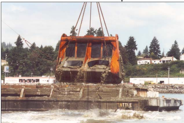
Dredging at PSNS with Environmental Bucket
