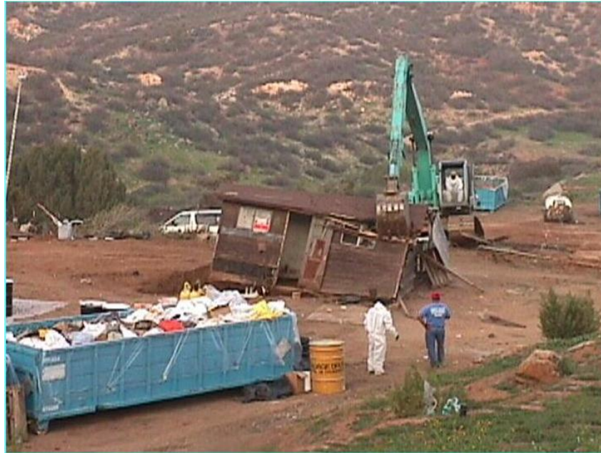
Knocking Over Shed to Get to Waste Below
