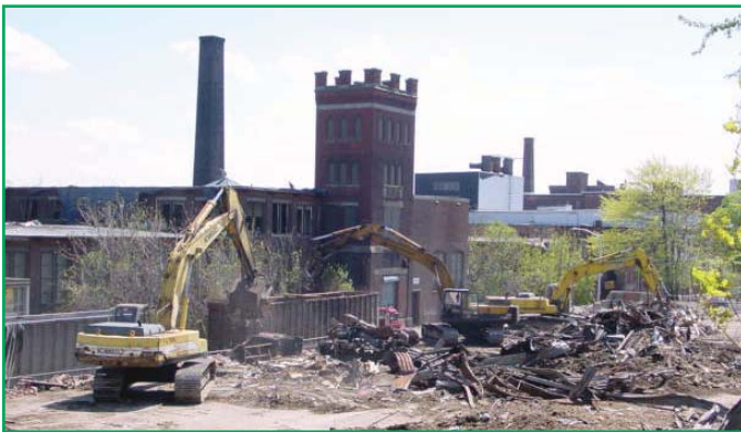
Recycling demolition material from the former industrial complex.
