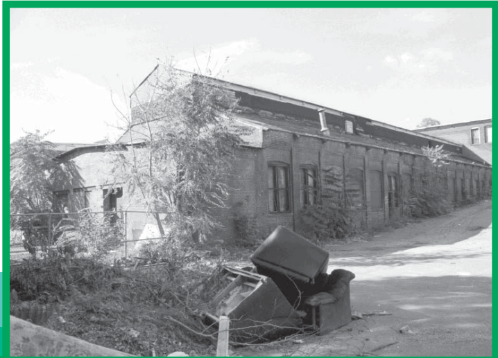
Abandoned industrial complex prior to cleanup and demolition activities.
